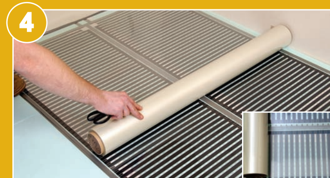
4 Cover the total ECOFILM PRO installation with POLYESTER VAPOUR BARRIER (available separately).
